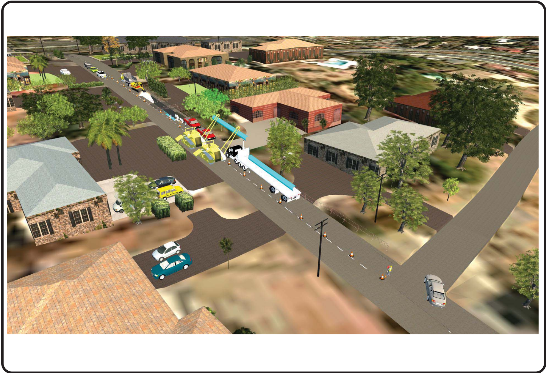
Figure 2.4-9: Typical Residential Construction – Temporary Road Closure
